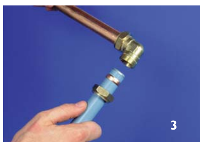
Ensure pipe is fully inserted
