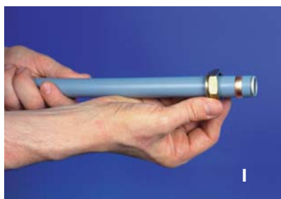
Insert support sleeve into pipe
