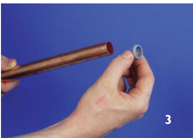
Insert copper end protector (HX61)
