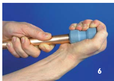
Tug back on the pipe to ensure grab wedge engages properly
